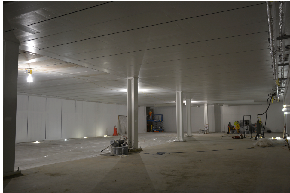
Tunnel warm and painted View inside linac tunnel from the west
