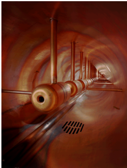
DTL tank Fermilab Room temperature drift tube linac
