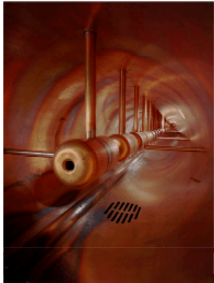
DTL tank - Fermilab
